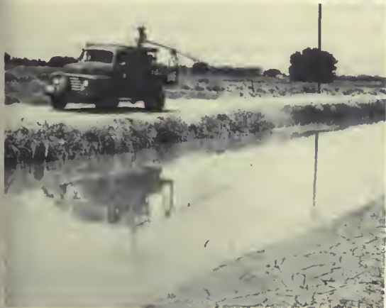
BUTANE-PROPANE burner clearing grass and weeds from lateral banks (at right). Below: Spraying weeds with fortified oil on Franklin Canal, Rio Grande project. Both photos by J. G. Koogler, Region 5.
